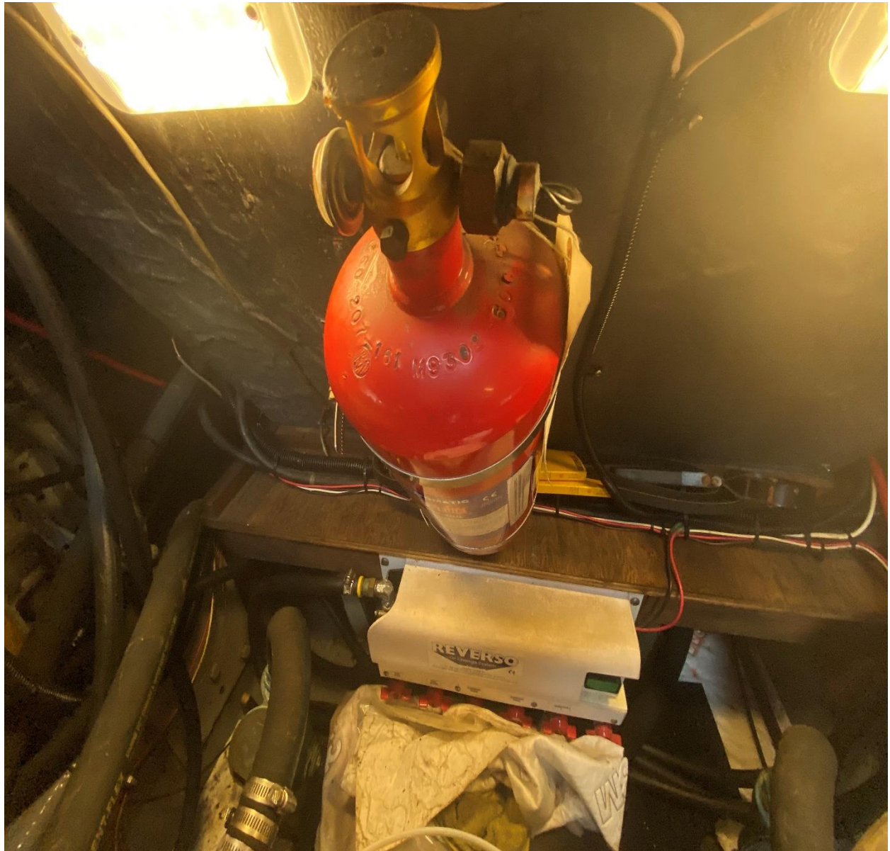
Engine Compartment Fire Suppression System
